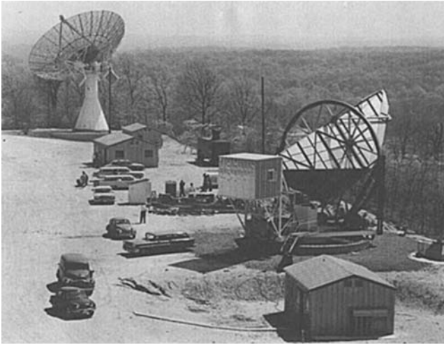
Fig. 4.9. The 20-ft “home-made” horn-reflector antenna in the foreground designed by A. B. Crawford (head of the Bell Labs department I joined in 1961) served as the Lab’s receiving station for Echo, the world’s first communications satellite project. Unlike this horn antenna, whose response pattern is tightly grouped about its main beam, the commercial 60-ft (diameter) parabolic antenna, shown in the background, picks up an appreciable amount of radiation from the ground, via spillover of the (downward-facing) feed horn located at its focus.
