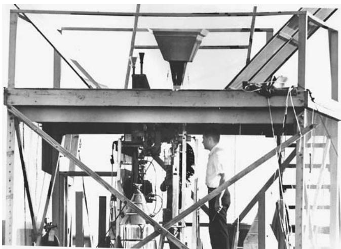
Fig. 4.22. The first Princeton CMBR experiment, on Guyot Hall. Peter Roll's outline appears behind the instrument; David Wilkinson is holding the screwdriver. Photo: Robert Matthews.
